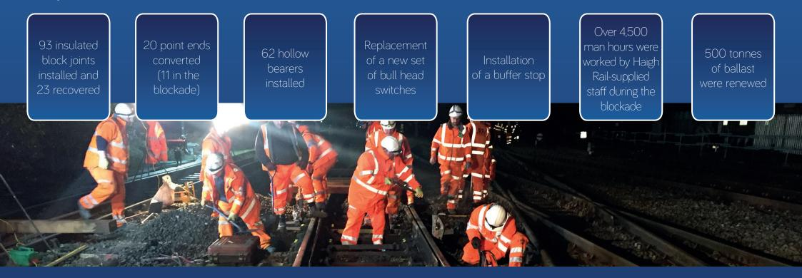
Haigh Rail was contracted through Network Rail and Siemens Rail Automation Holdings to provide a range of works for the re-signalling project at Gresty Lane in Crewe (GRIP 5-8). The works were successfully commissioned during the nine-day blockade.
