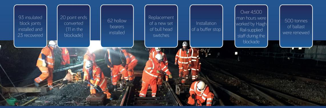
Haigh Rail was contracted through Network Rail and Siemens Rail Automation Holdings to provide a range of works for the re-signalling project at Gresty Lane in Crewe (GRIP 5-8). The works were successfully commissioned during the nine-day blockade.
