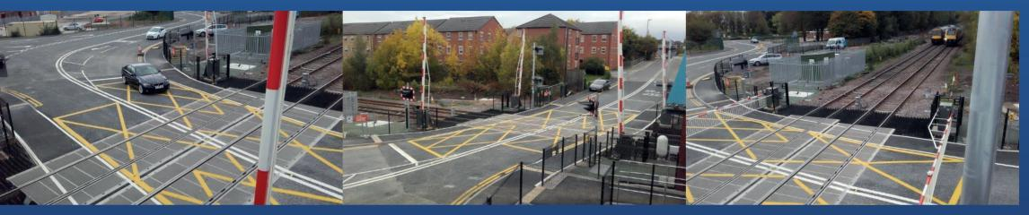
Spondon Level Crossing was a unique job that Haigh Rail recently undertook on behalf of partner Siemens Rail Automation. The works consisted of a full level crossing deck renewal, plus realignment of the existing footprint to accommodate a new alignment of the highway.
